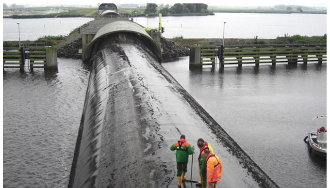
Ramspol barrier closed, The Netherlands
