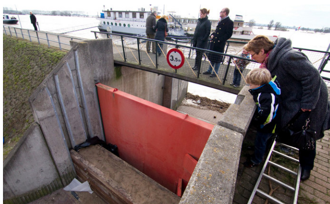
Coupure in existing walls
