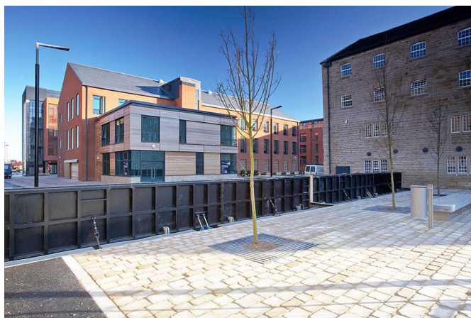
Flipable flood barrier, Wakefield (UK)
