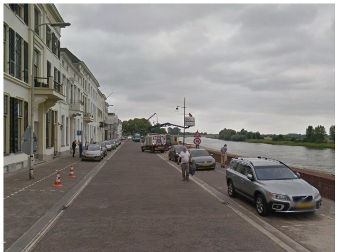
Low wall as part of the street profile and primary flooddefence. IJsselkade Zutphen
