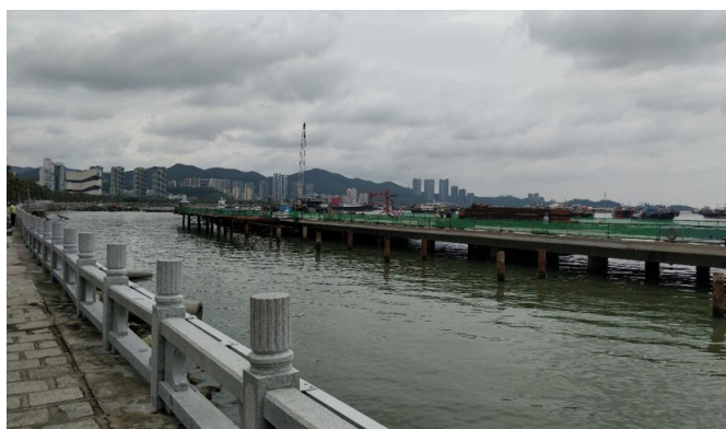
Off-shore construction close to the quay
