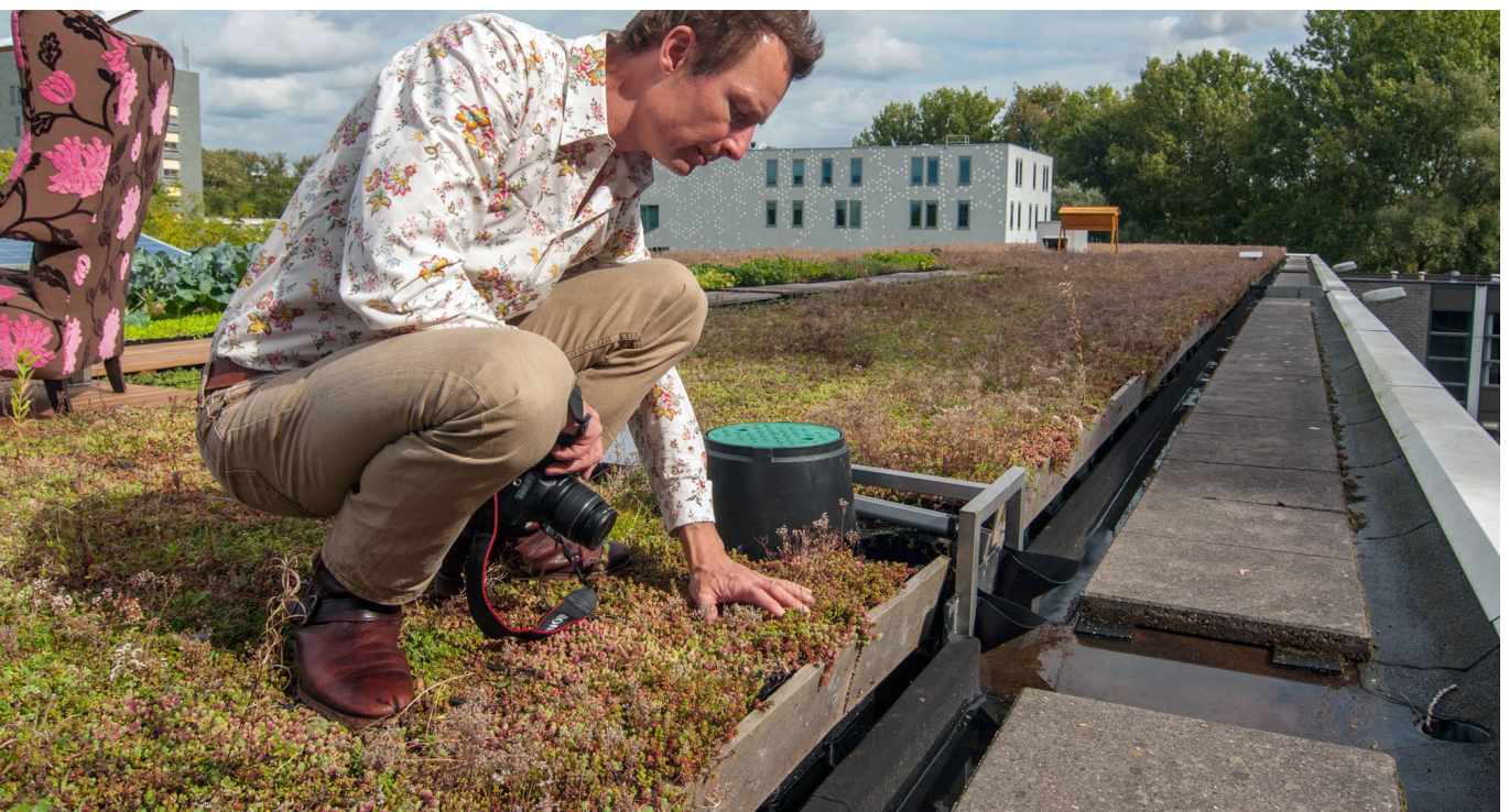
Figure 10: A Blue-Green (retention) roof in Amsterdam to increase the sponge effect of the city.
