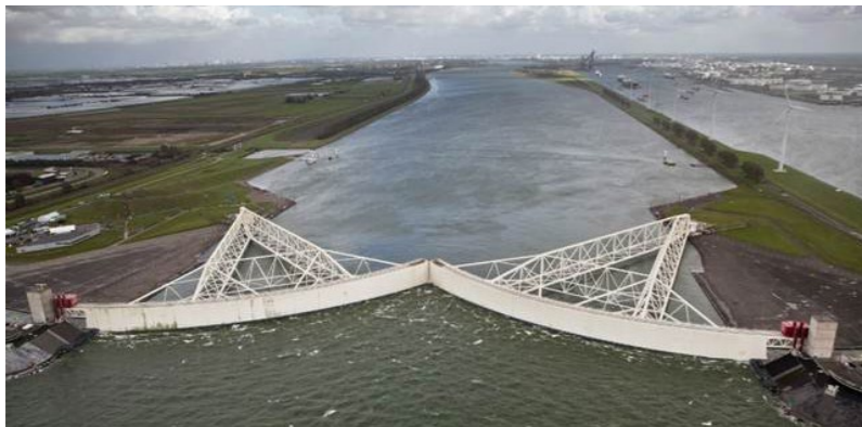
Flood gates, infrastructure, Europoort Rotterdam (NL)
