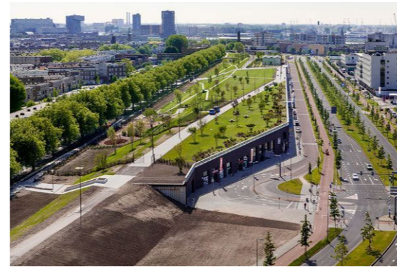
Delay, water storage, Roofpark, Rotterdam
