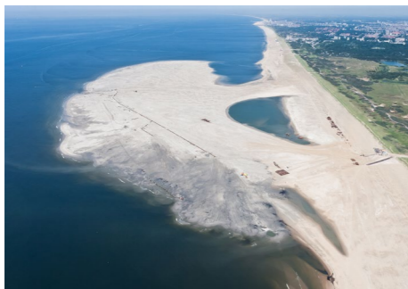
Sand engine, provoke sedimentation, The Hague (NL)
