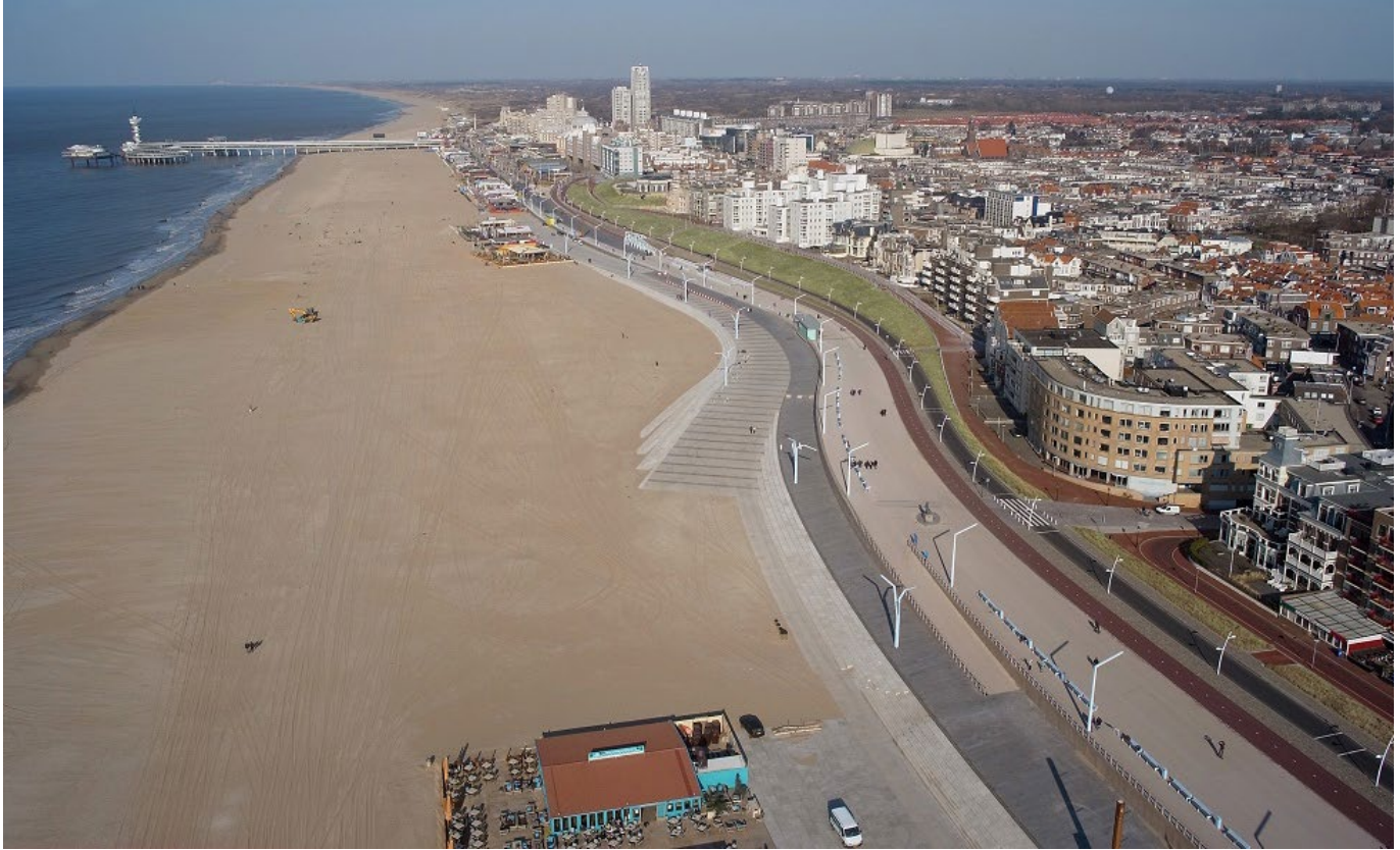
Overview of the new coastal defence which acts as a public space as well
