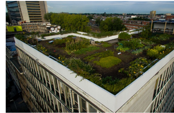
Delay, water storage, roof garden, agriculture, Rotterdam
