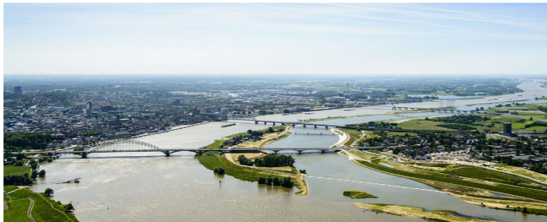
Room for the river, ecology, dynamic landscape, Nijmegen (NL)
